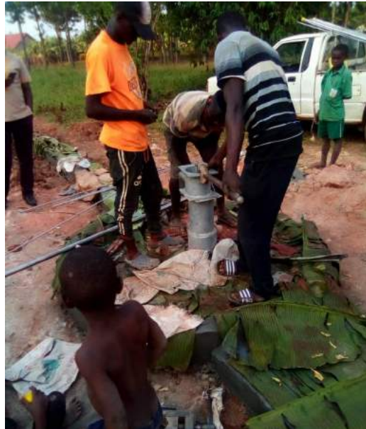
Figure 12: Installation of ground water well. (Whatsapp Communication)
