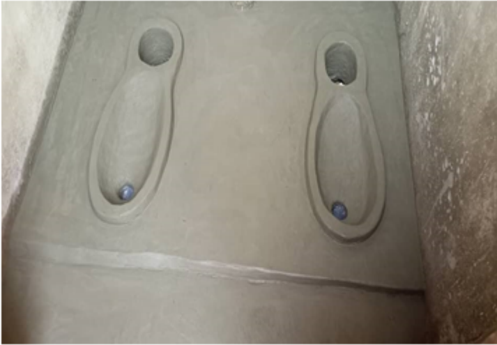
Figure 4: An example of ECOSAN separation pans moulded with mortar.
